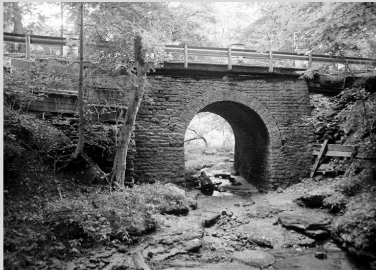
View of culvert, looking north-northeast, 2006. (Douglas Bailey)
