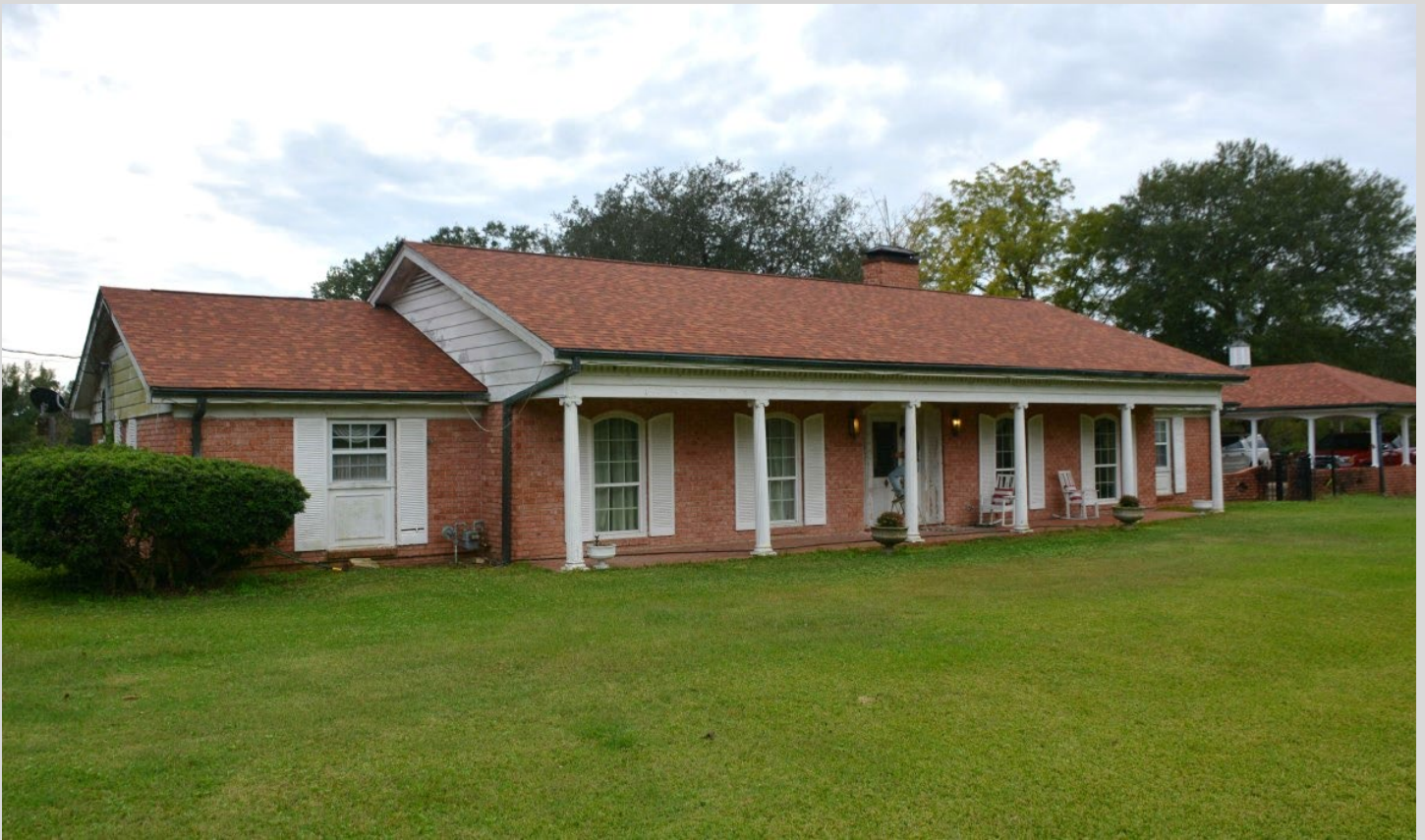
Attwood House, north façade, 2022. (Ralph Wilcox)
