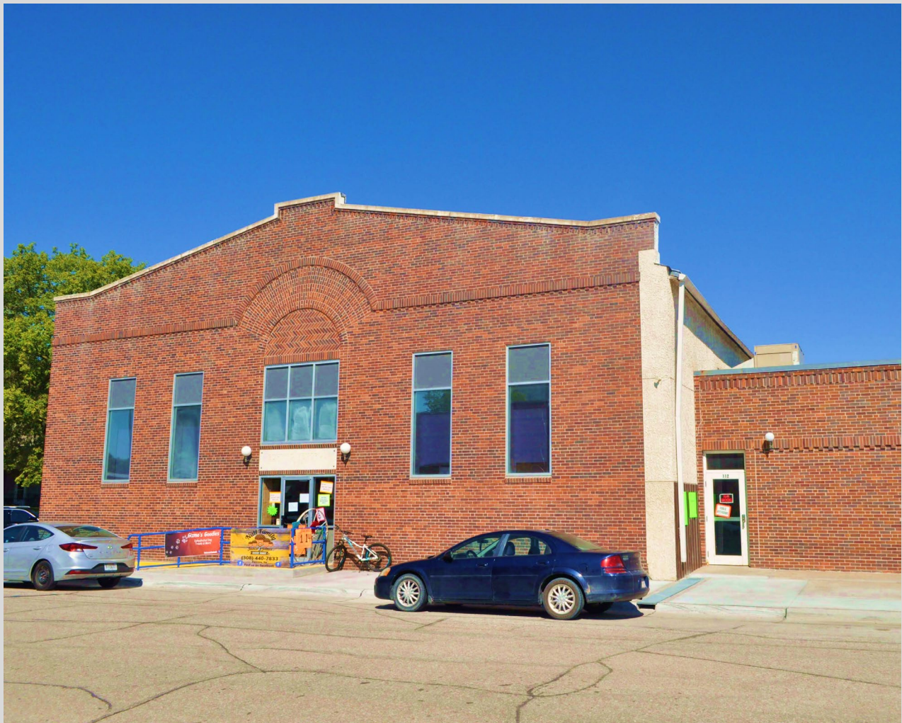
Bohning Memorial Auditorium, main elevation, view facing northwest. (Patrick Haynes)
